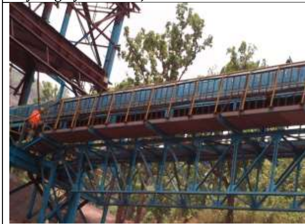
Covering of Conveyor from JH-2 to JH-3 by erecting FRP conveyor hood.
